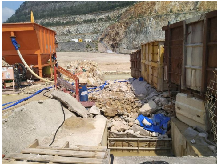
Q3: Wastewater treatment facility 110 cu. m. + AquaSed of 60 cu. m. per hour
