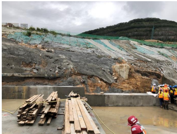
Exposed surface was covered by cement motar
