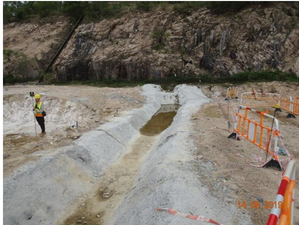
Perimeter channel to collect site surface
