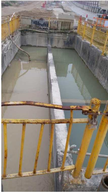
Q6: Wastewater treatment facility 24 cu. m.
